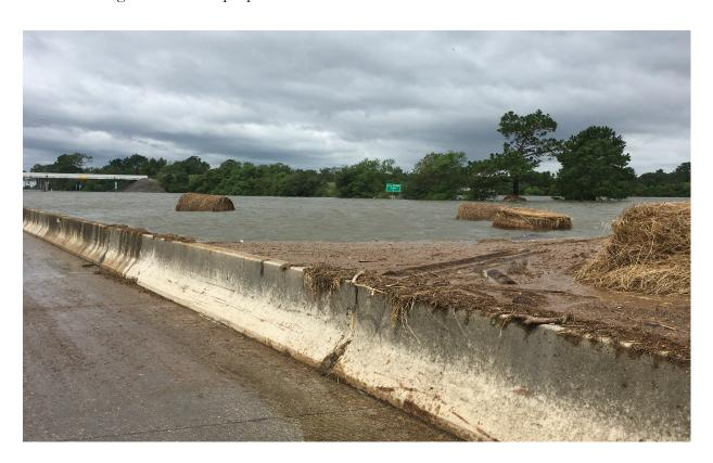
25. Likewise, in September 2019, TxDOT's median barrier/dam along IH-10 blocked rainfall runoff from overtopping the roadway during and after Tropical Storm Imelda. Again, eastbound traffic lanes remained open and conferred a benefit to the public at large. And, again, the blocked storm runoff water backed up and flooded and severely damaged Plaintiffs' property.
