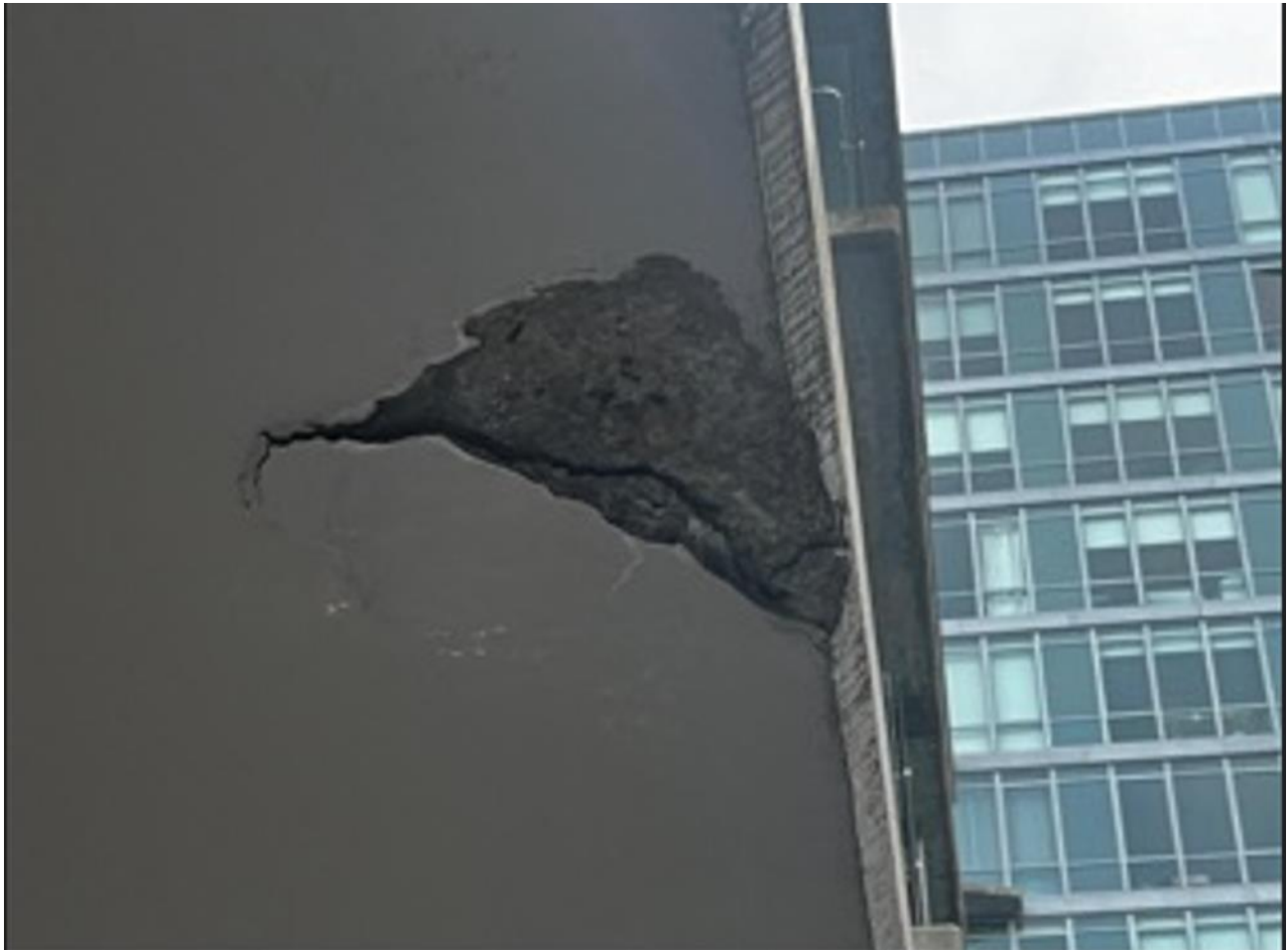
Figure 6 Cracked Balcony
