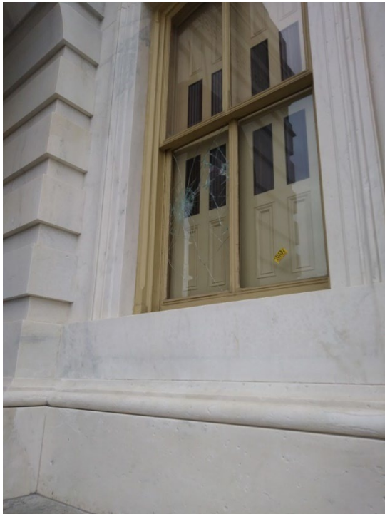
Figure 11 – Baugham cellphone photograph taken after exiting the Capitol Building
