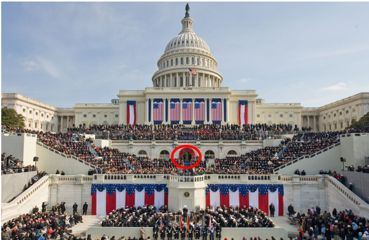
Image 1 (Lower West Terrace tunnel entrance)
