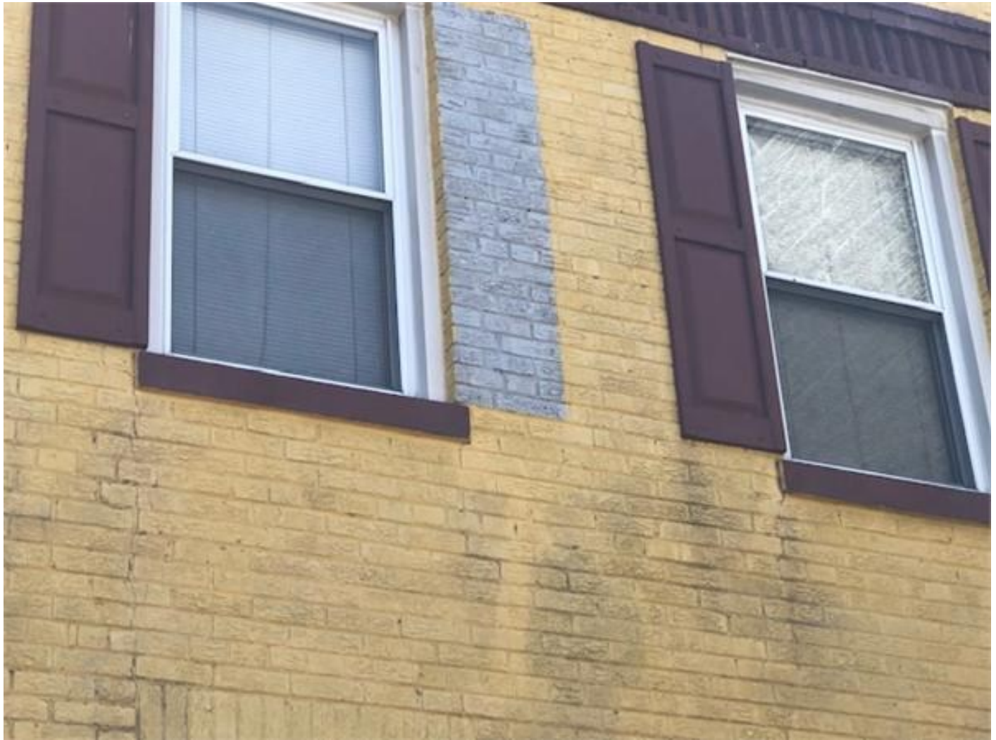
Fig 9. 770 Princeton Pl. NW@ Front underpinned wall.
