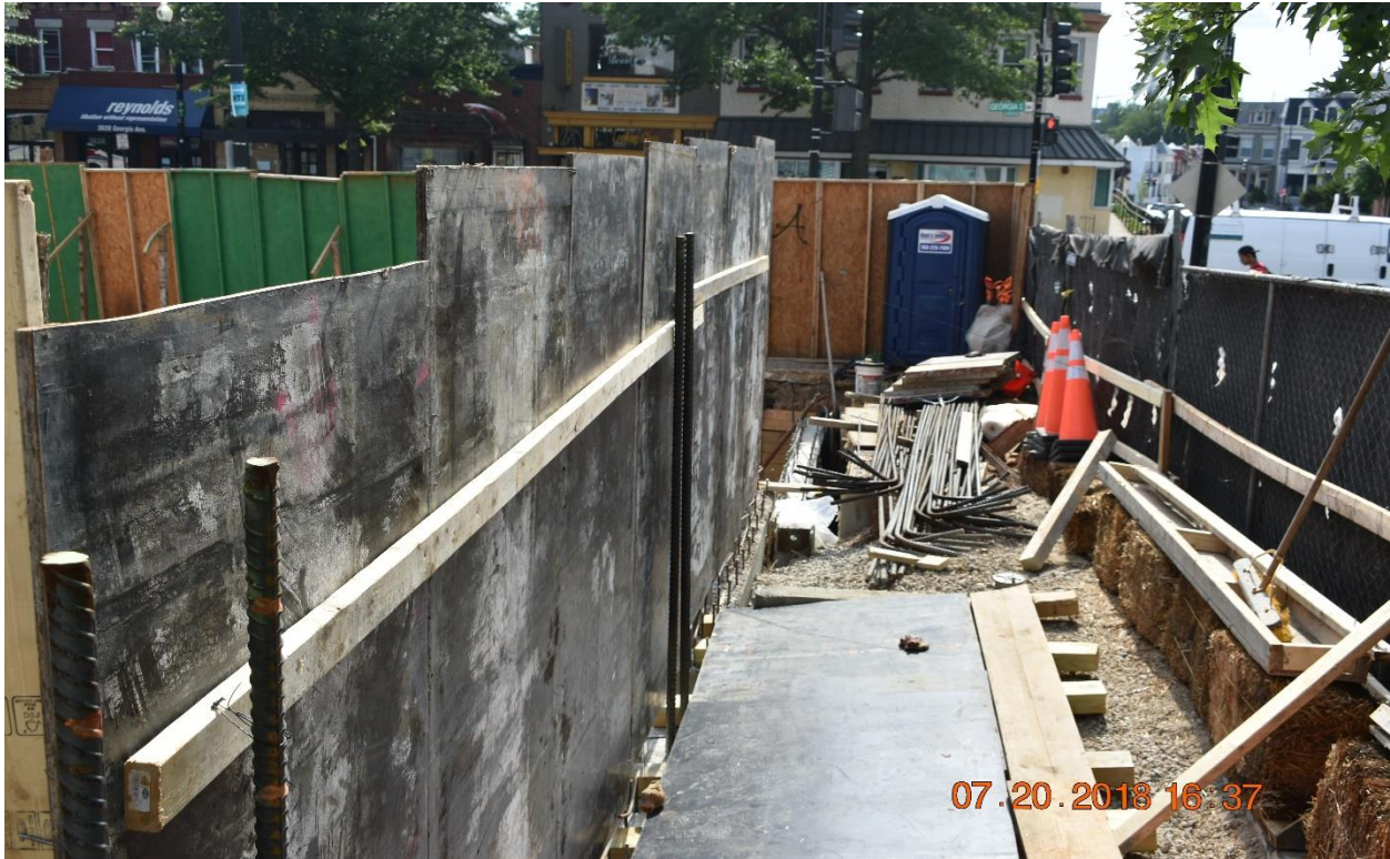
New foundation wall on Princeton Place/sidewalk supported
