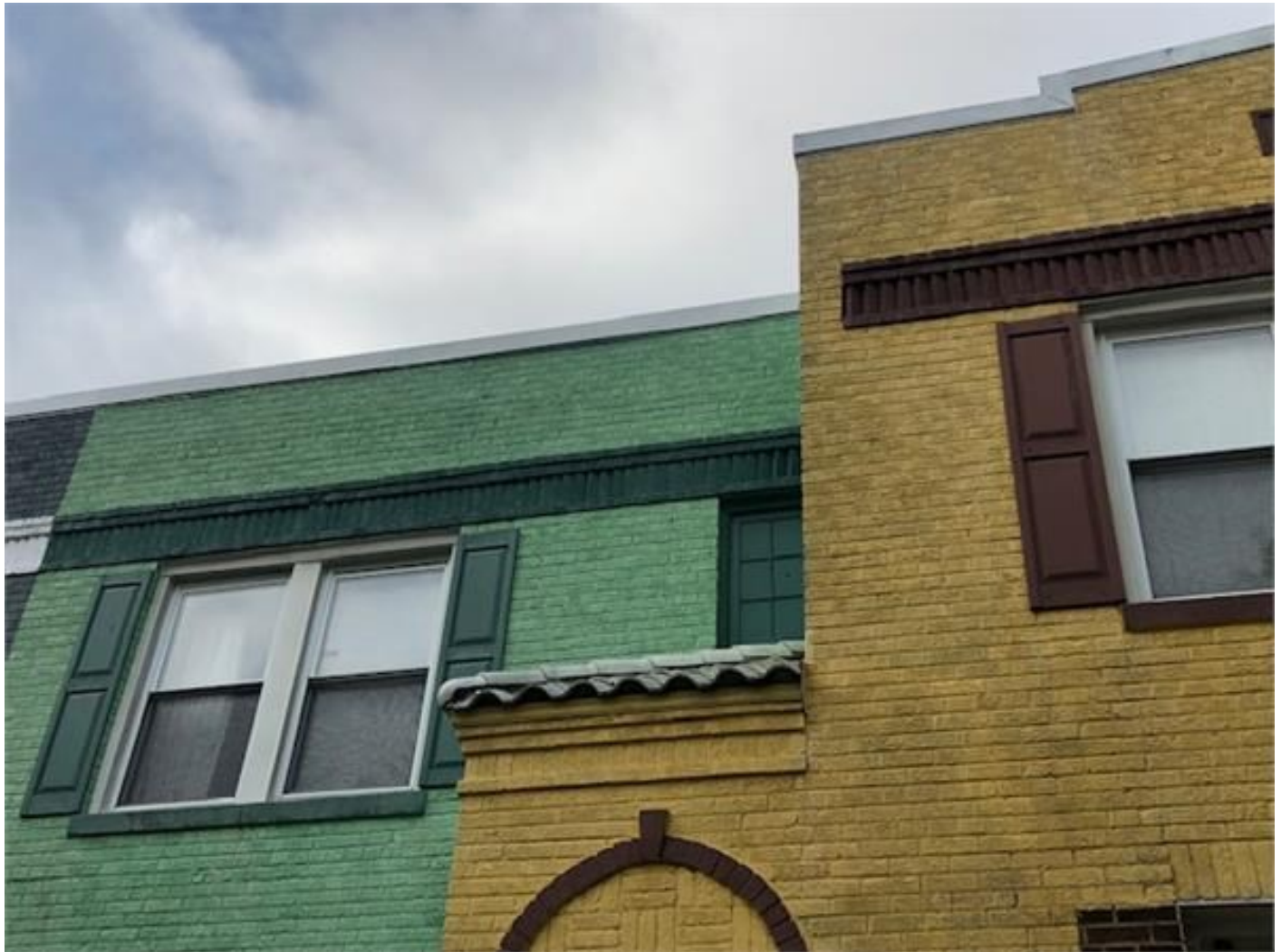
Fig 6. 770 Princeton Pl. NW@ Front underpinned wall.
