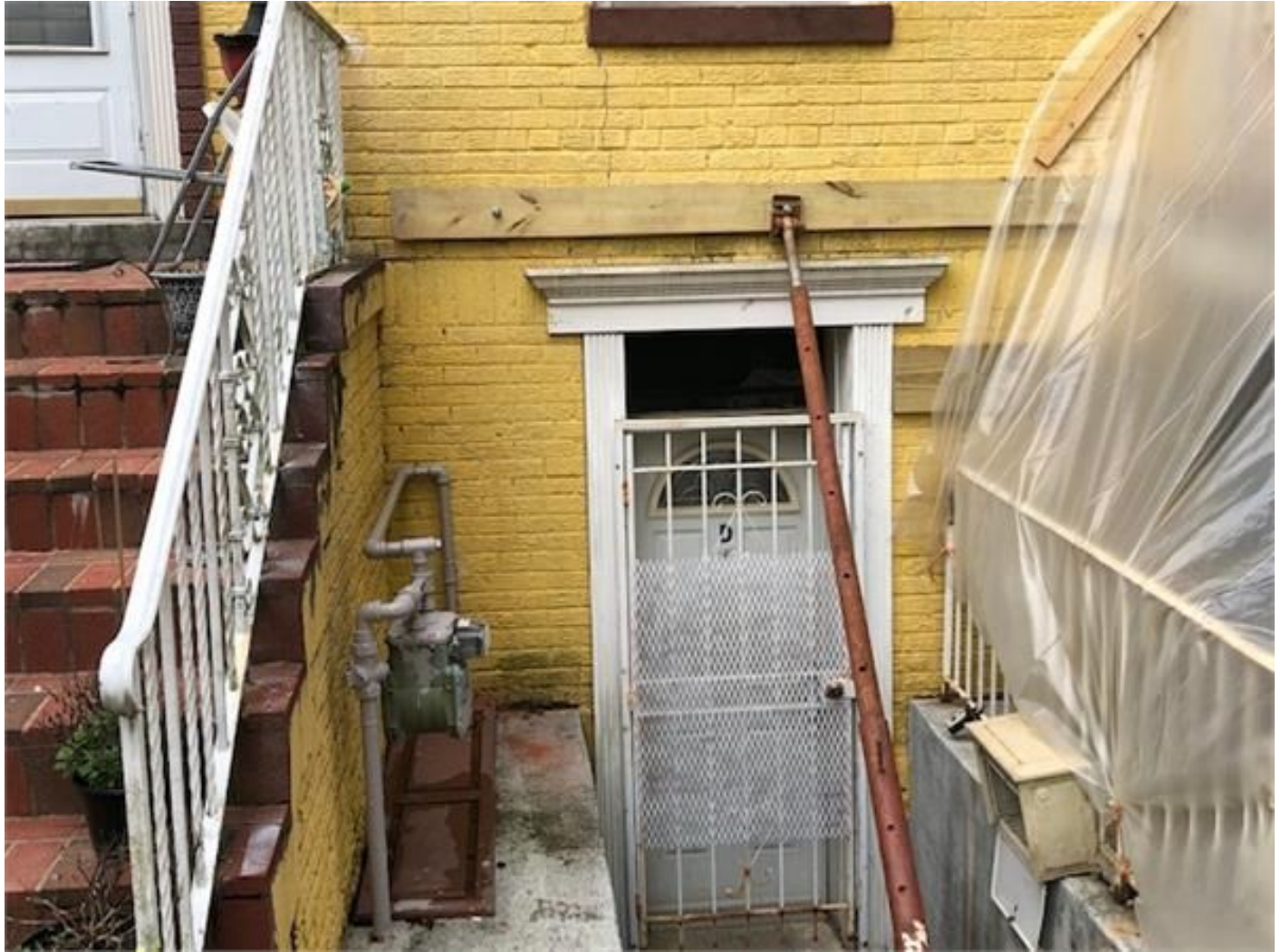
Fig 1. 770 Princeton Pl. NW@ Front underpinned wall.
