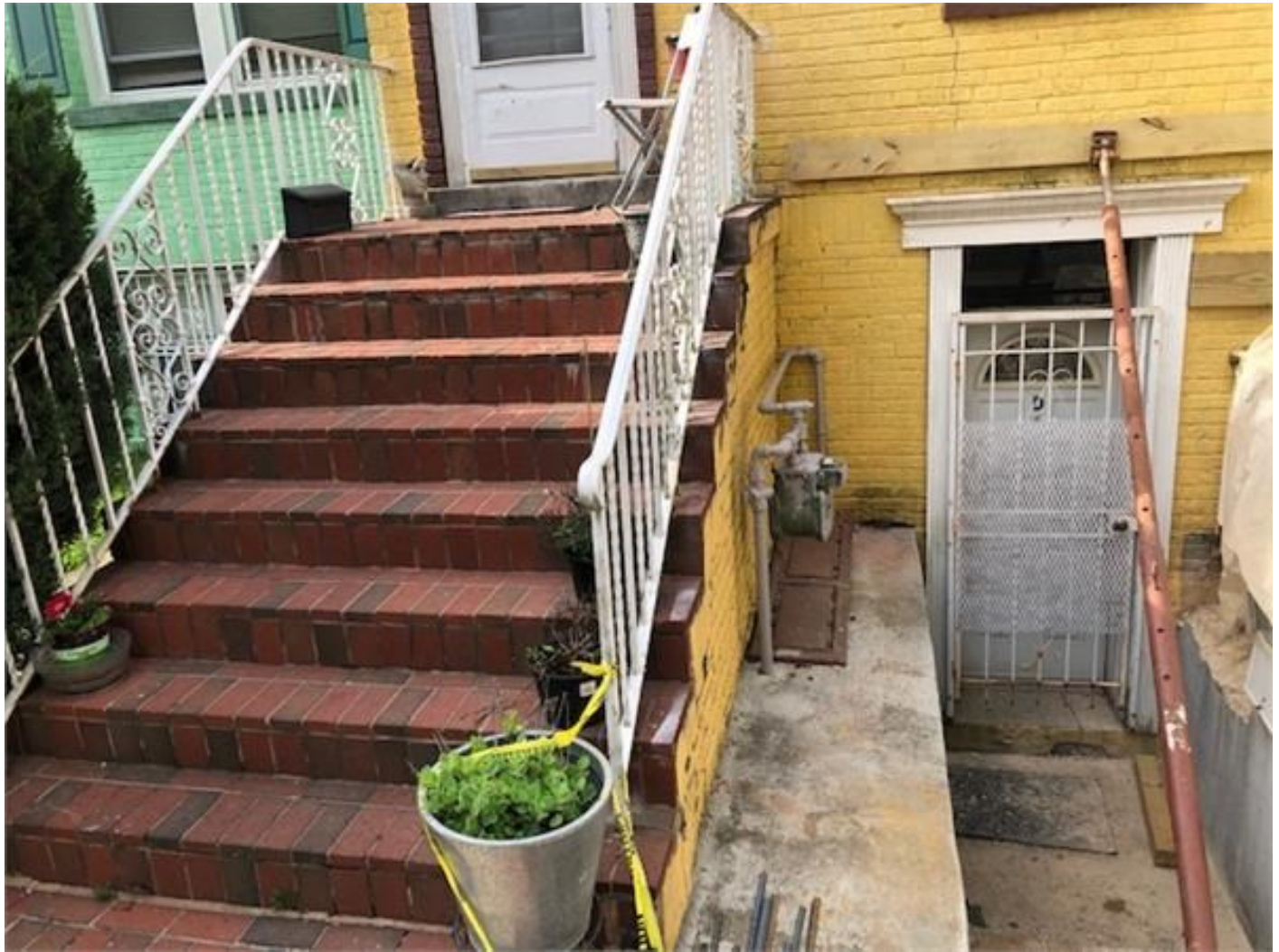
Fig 10. 770 Princeton Pl. NW@ Front underpinned wall.
