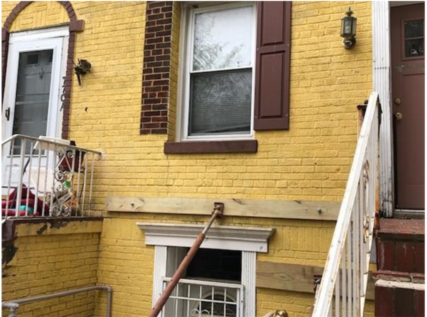
Fig 2. 770 Princeton Pl. NW@ Front underpinned wall.
