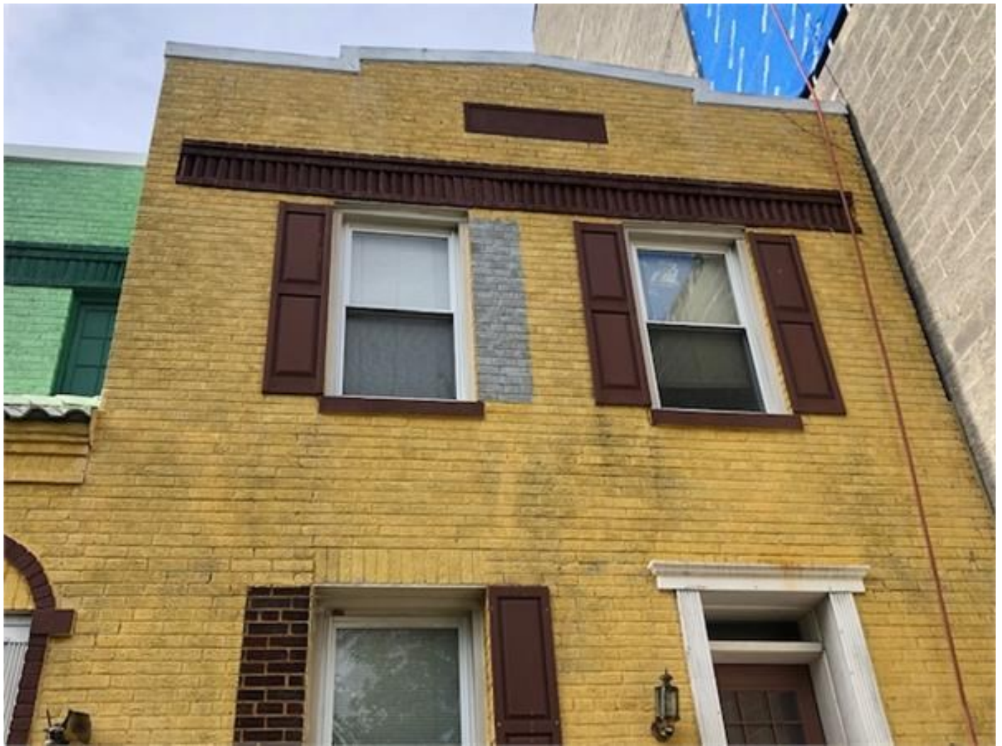
Fig 3. 770 Princeton Pl. NW@ Front Underpinned Wall
