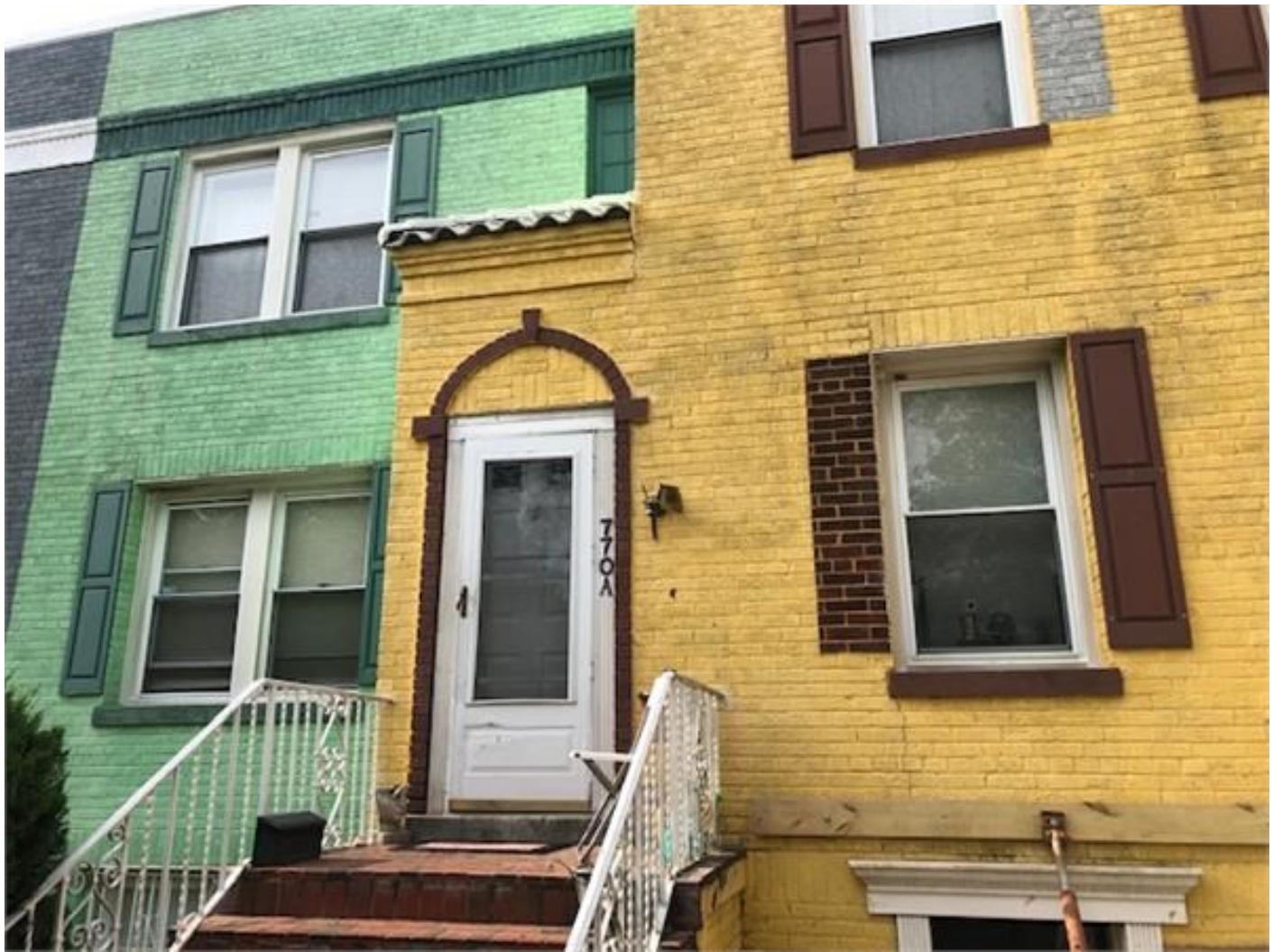
Fig 2. 770 Princeton Pl. NW@ Front underpinned wall.
