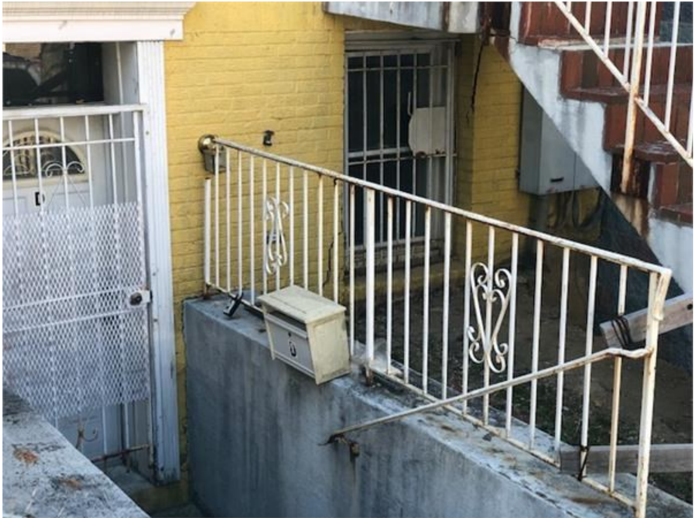
Fig 10. 770 Princeton PI. NW@ Front underpinned wall.
