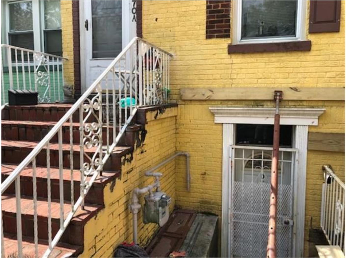
Fig 1. 770 Princeton PI. NW@ Front underpinned wall.
