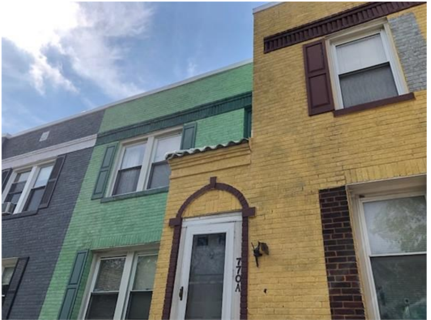
Fig 7. 770 Princeton Pl. NW@ Front underpinned wall.
