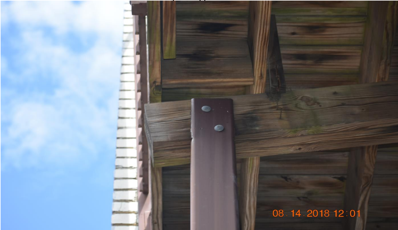
Rear deck post support on 8/14/2018
