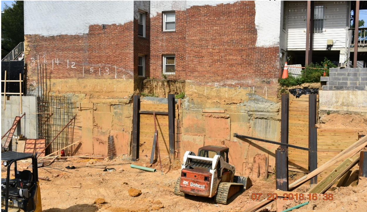
Lateral support of underpinning and shoring system
