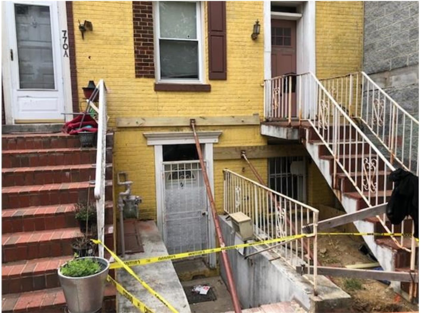
Fig 10. 770 Princeton Pl. NW@ Front underpinned wall.
