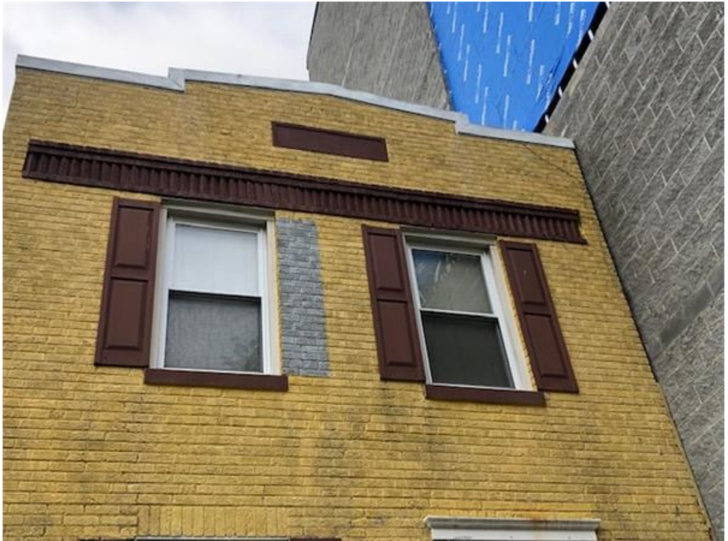
Fig 3. 770 Princeton Pl. NW@ Front Underpinned Wall
