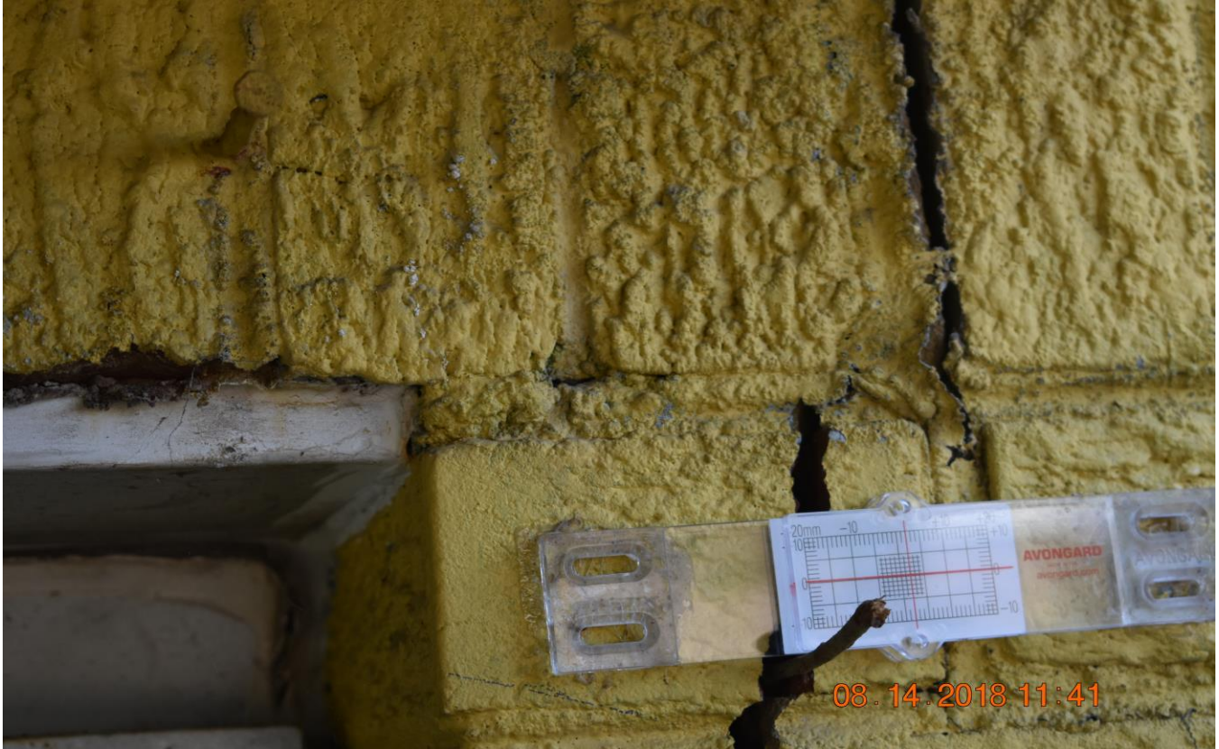
Monitor on right window corner of building façade wall (Taken 8/14/2018).
