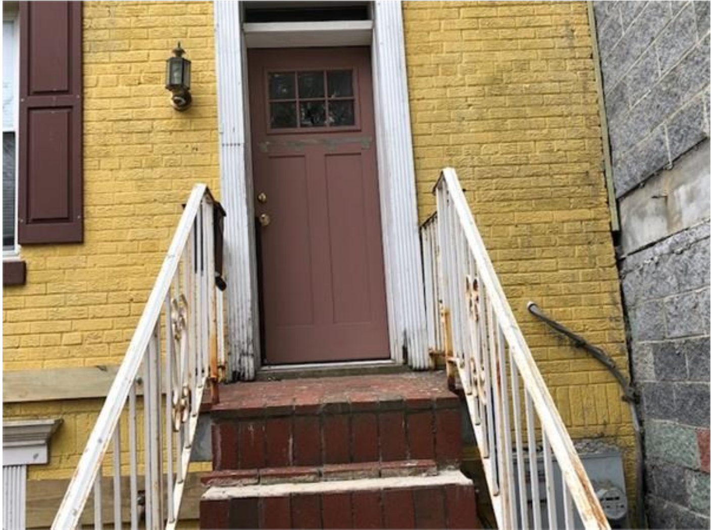
Fig 1. 770 Princeton Pl. NW@ Front underpinned wall.
