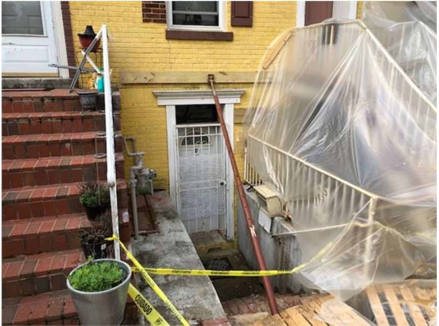
Fig 7. 770 Princeton Pl. NW@ Front underpinned wall.
