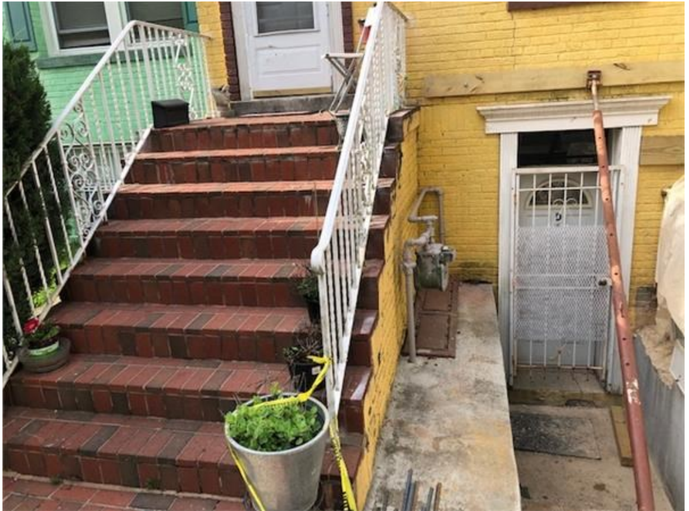
Fig 7. 770 Princeton Pl. NW@ Front underpinned wall.
