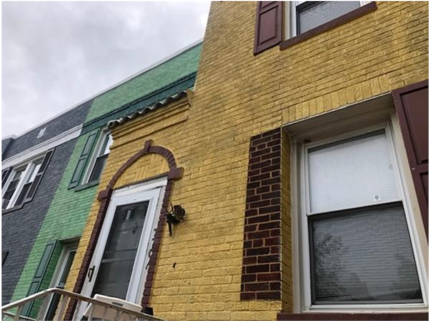
Fig 6. 770 Princeton Pl. NW@ Front underpinned wall.
