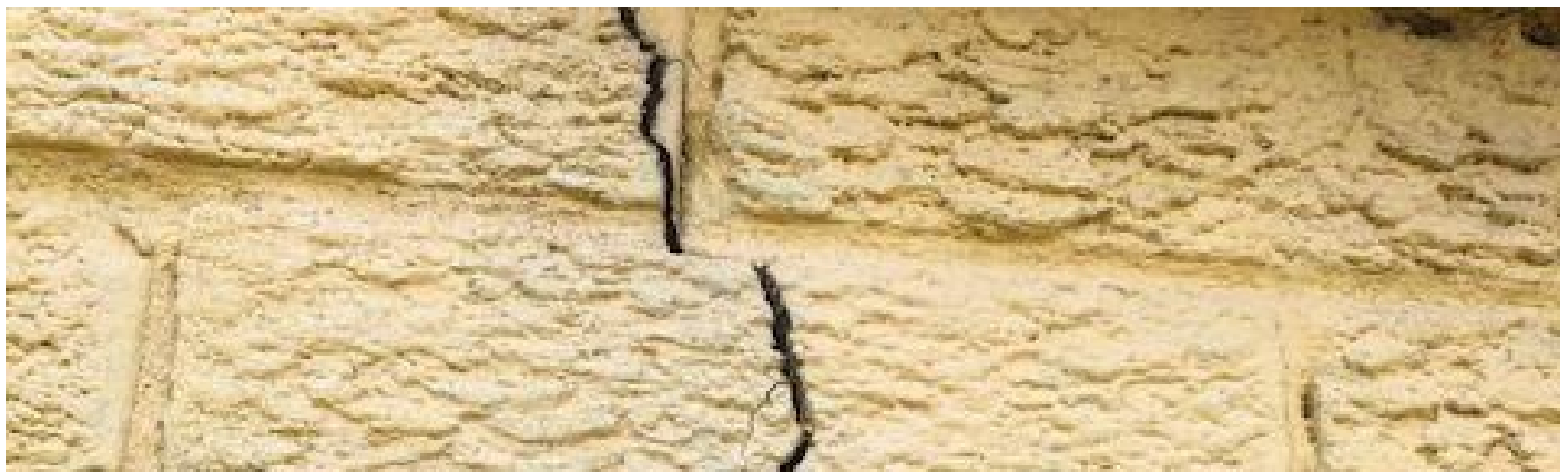
Fig 2. 770 Princeton Pl. NW@ Front underpinned wall.
