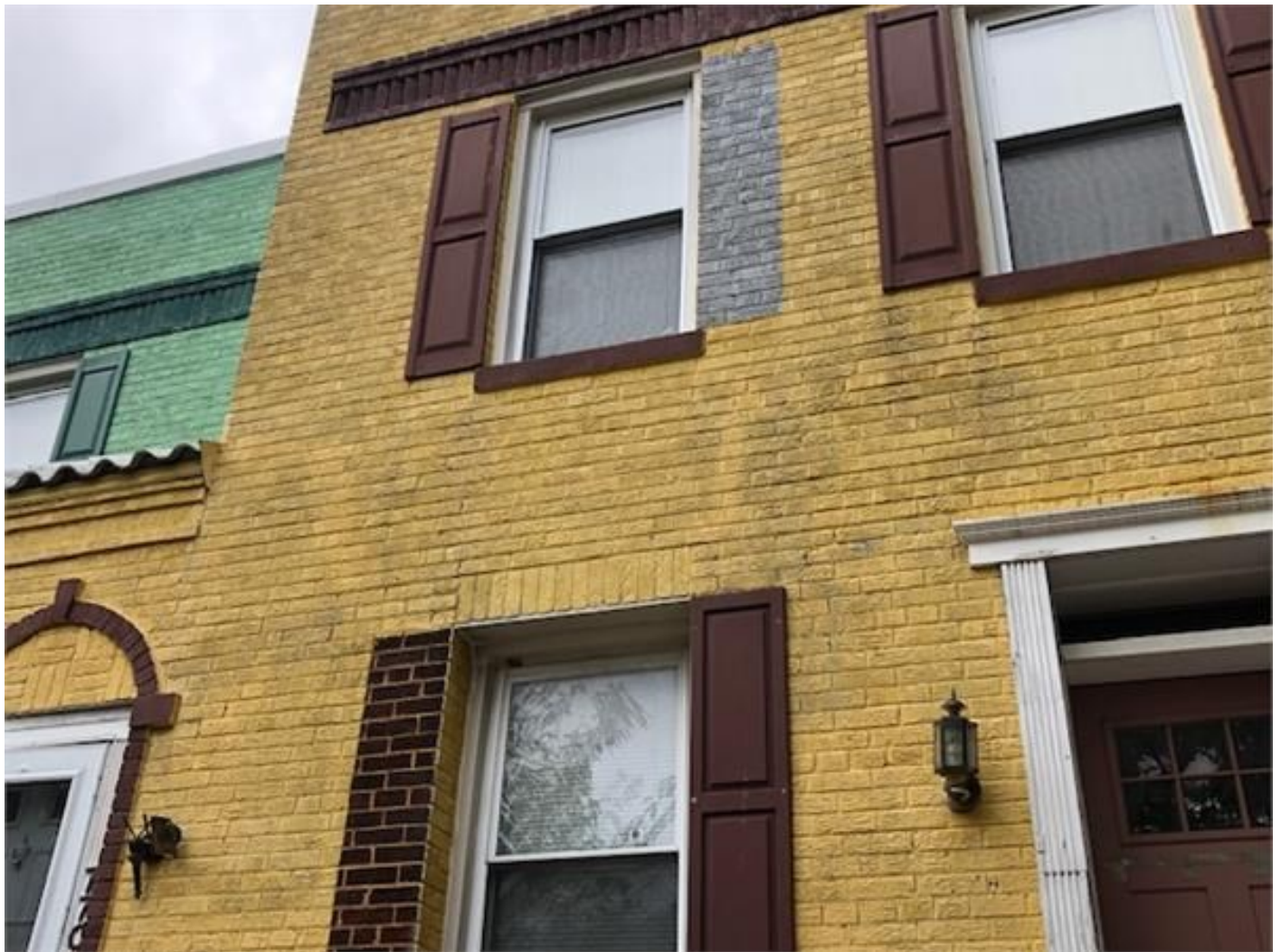
Fig 3. 770 Princeton Pl. NW@ Front Underpinned Wall
