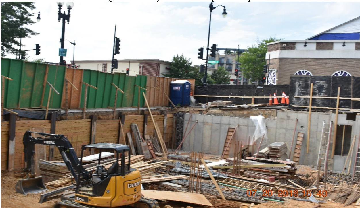
Bracing of newly poured wall.
