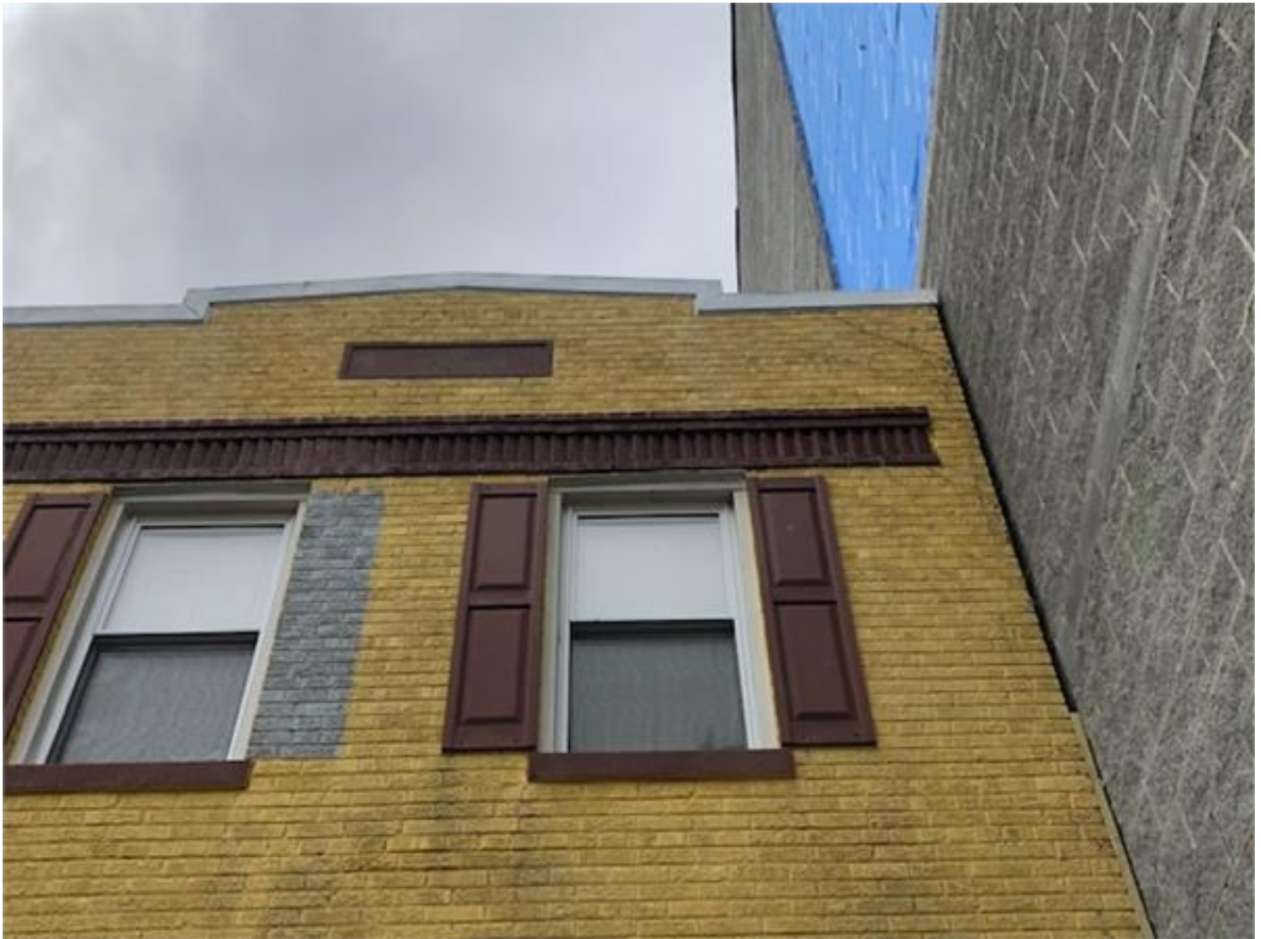
Fig 4. 770 Princeton Pl. NW@ Front underpinned wall.
