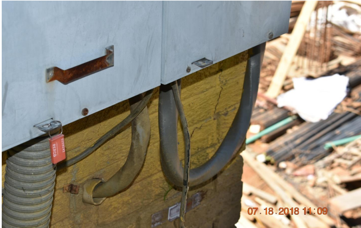
Crack monitor installed
