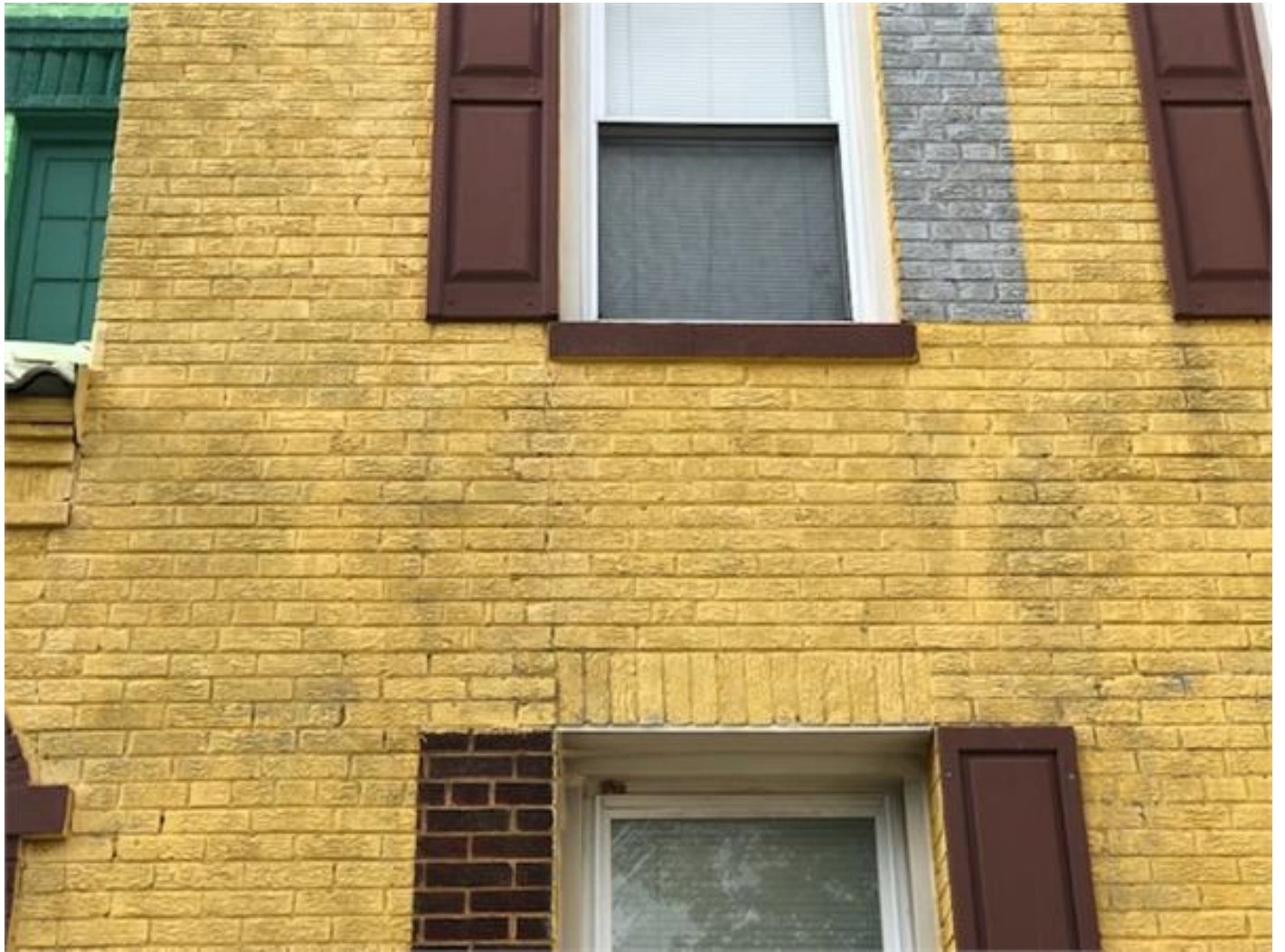
Fig 4. 770 Princeton Pl. NW@ Front underpinned wall.
