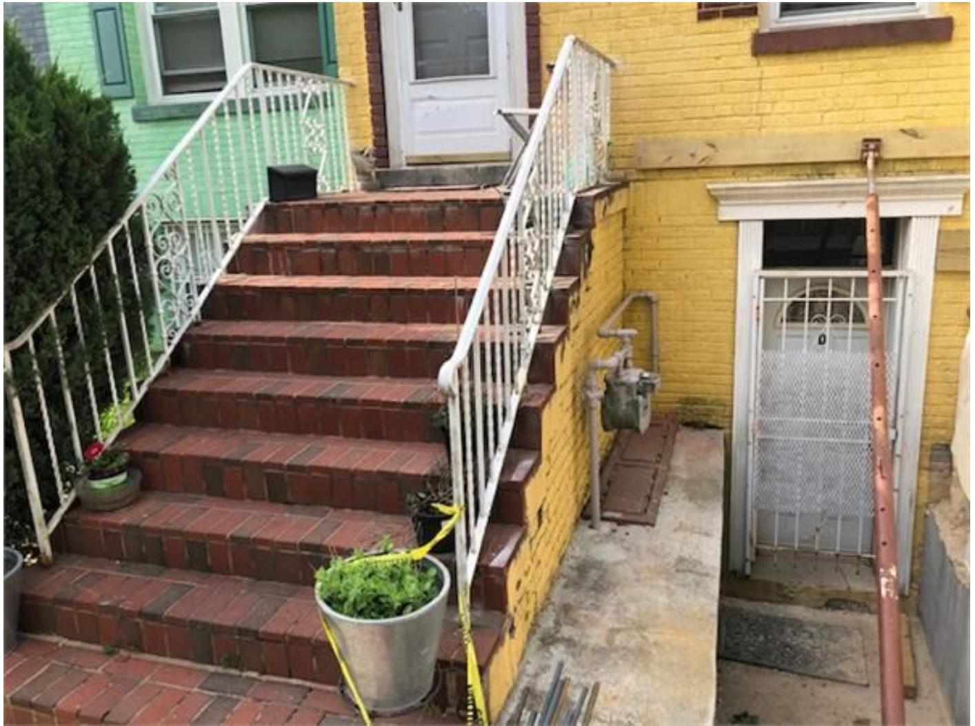
Fig 1. 770 Princeton Pl. NW@ Front underpinned wall.
