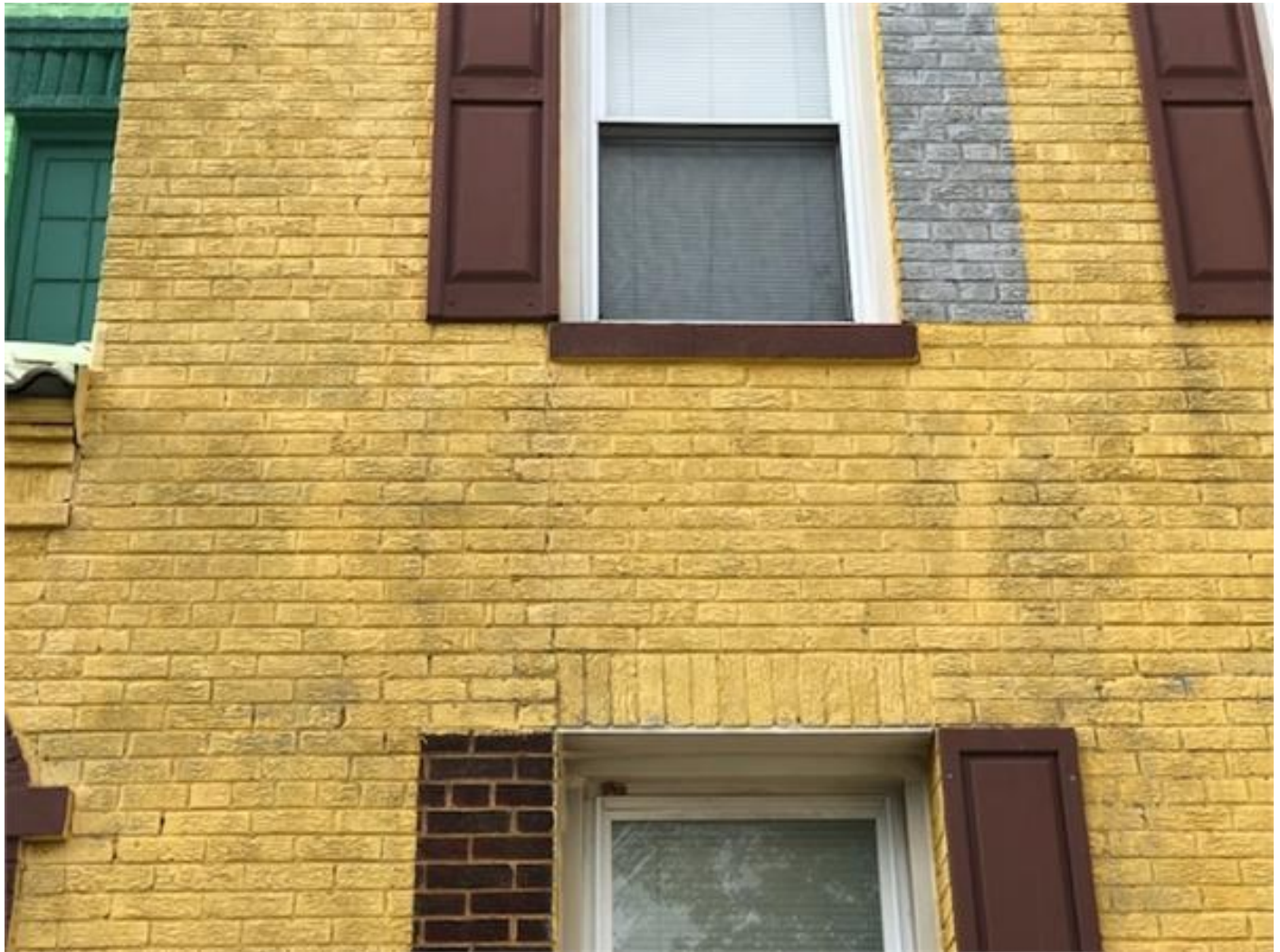
Fig 8. 770 Princeton Pl. NW@ Front underpinned wall.
