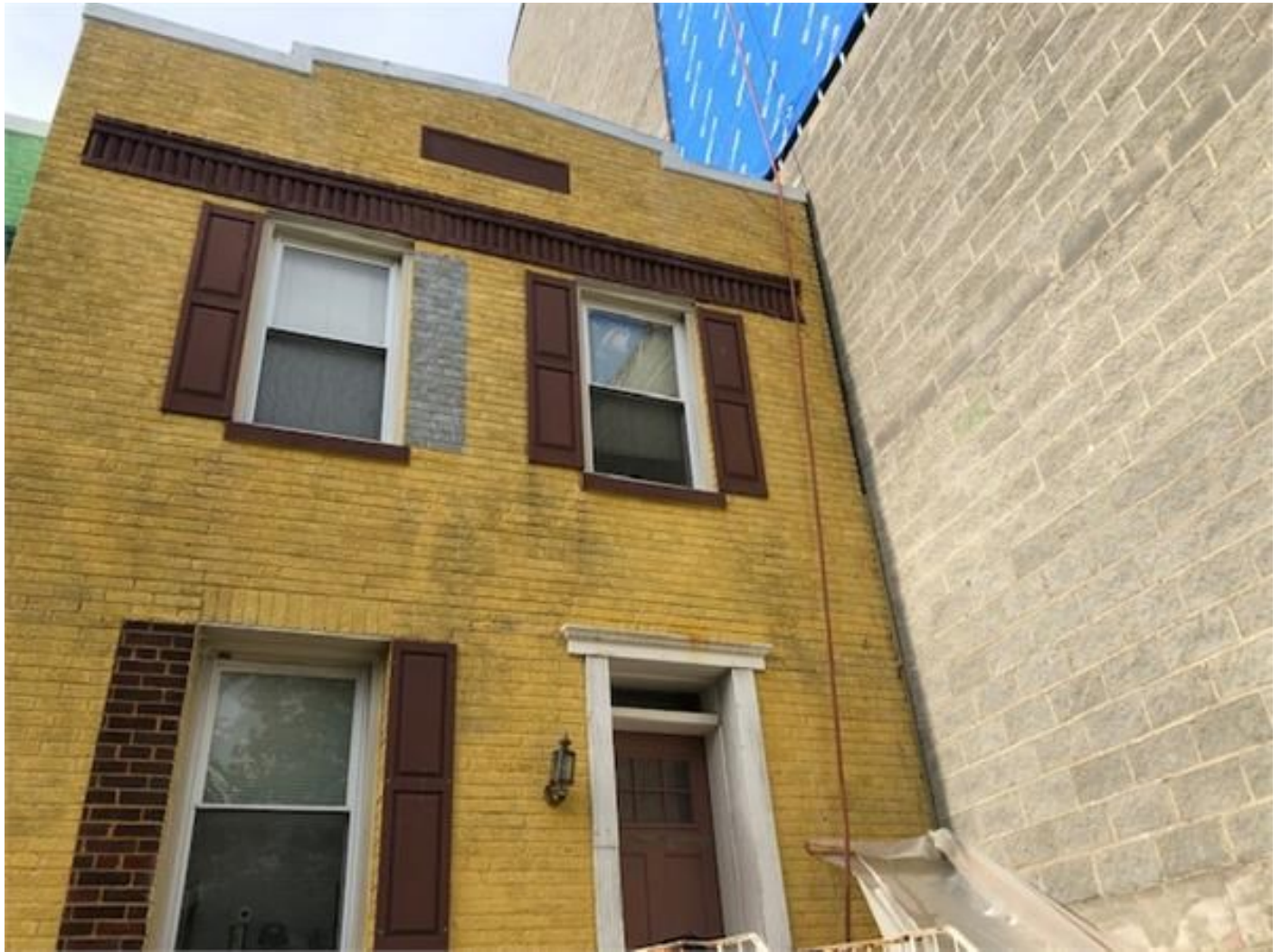
Fig 9. 770 Princeton Pl. NW@ Front underpinned wall.
