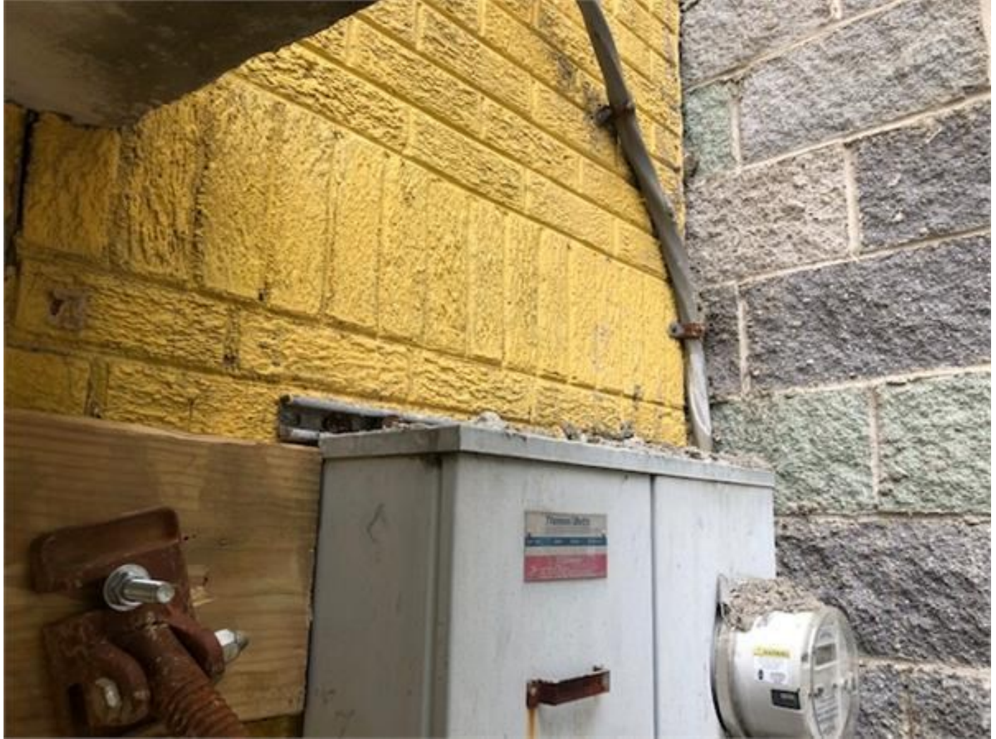
Fig 9. 770 Princeton Pl. NW@ Front underpinned wall.
