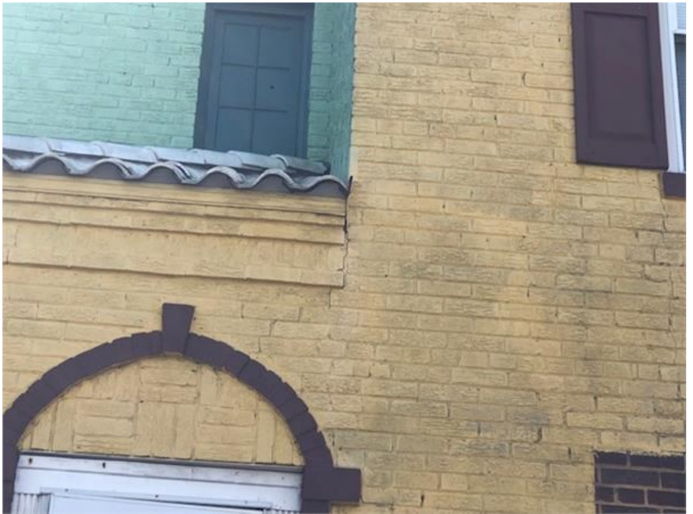
Fig 8. 770 Princeton Pl. NW@ Front underpinned wall.
