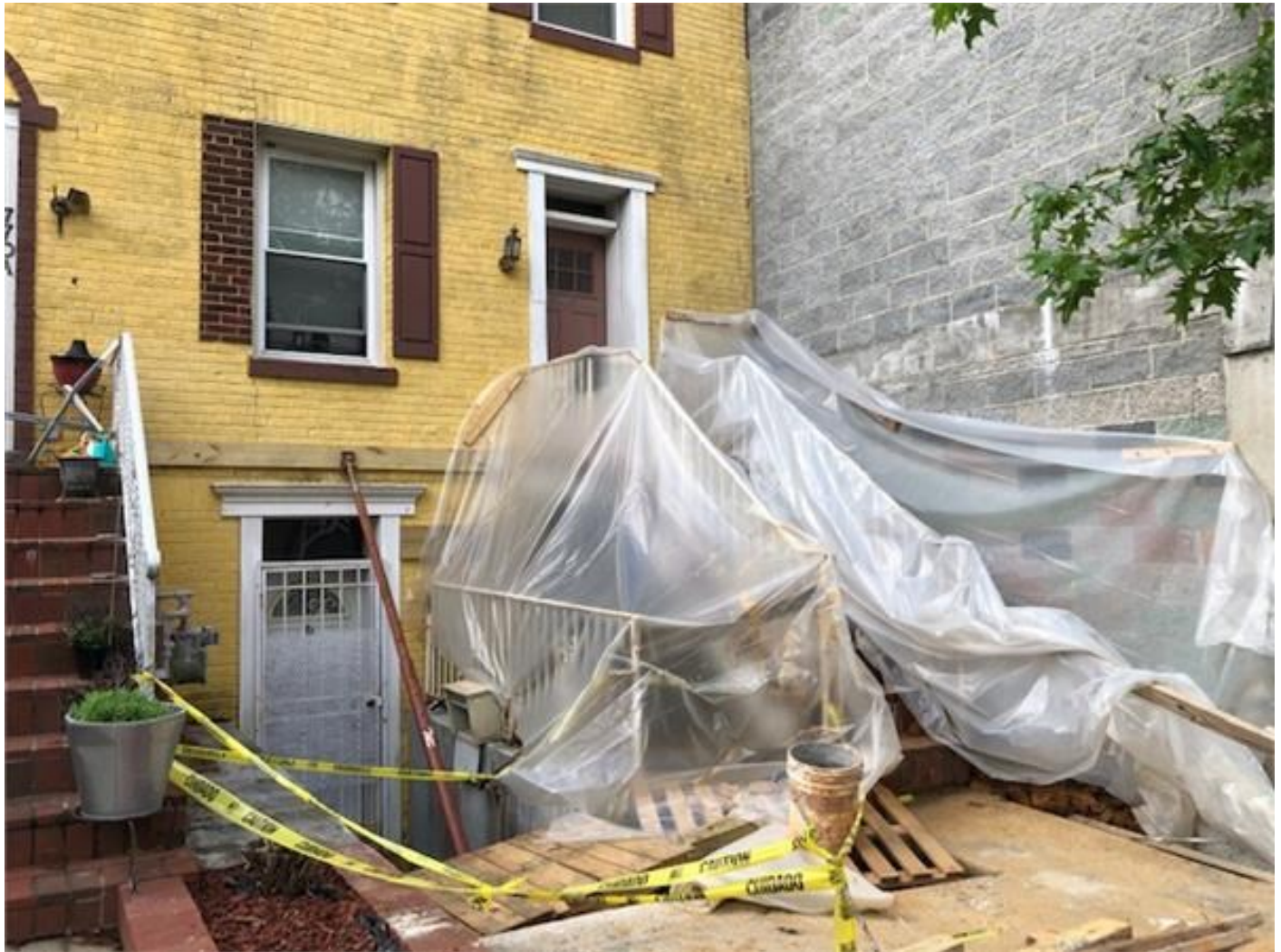
Fig 10. 770 Princeton Pl. NW@ Front underpinned wall.
