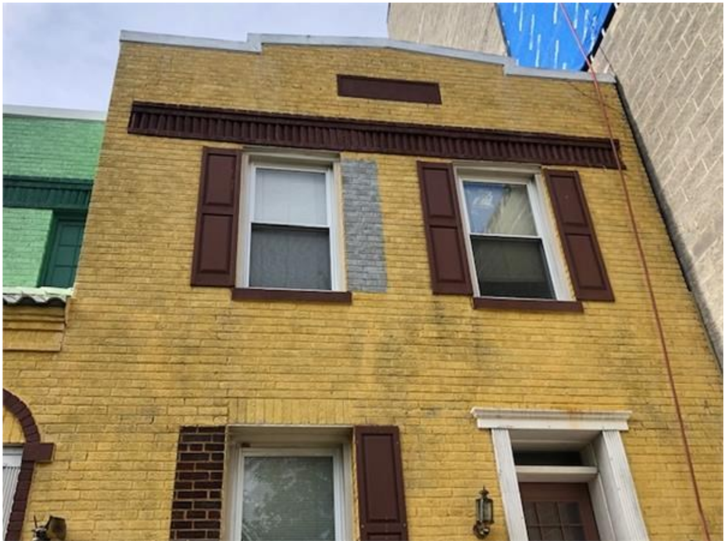
Fig 3. 770 Princeton Pl. NW@ Front Underpinned Wall
