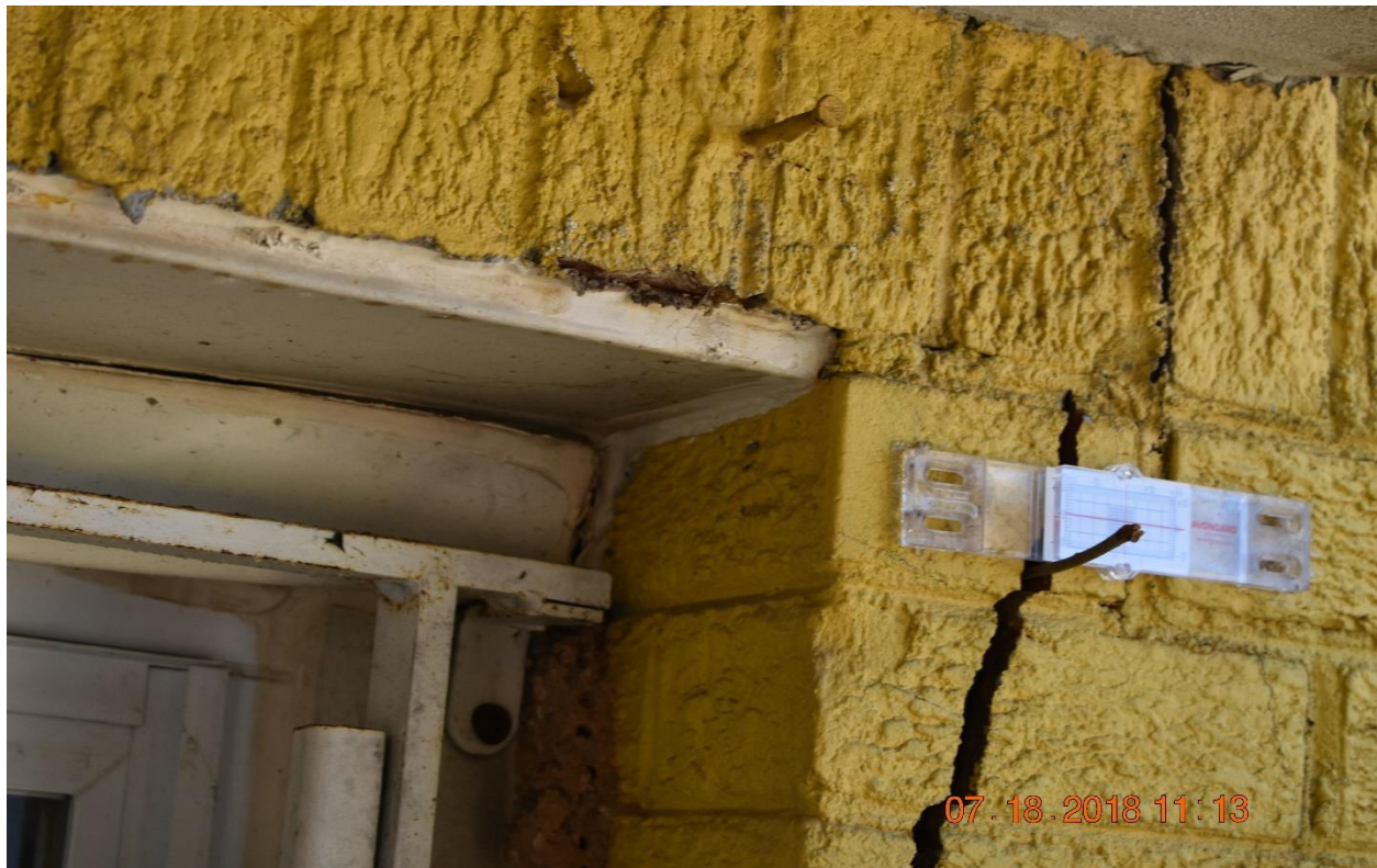
Crack monitor installed
