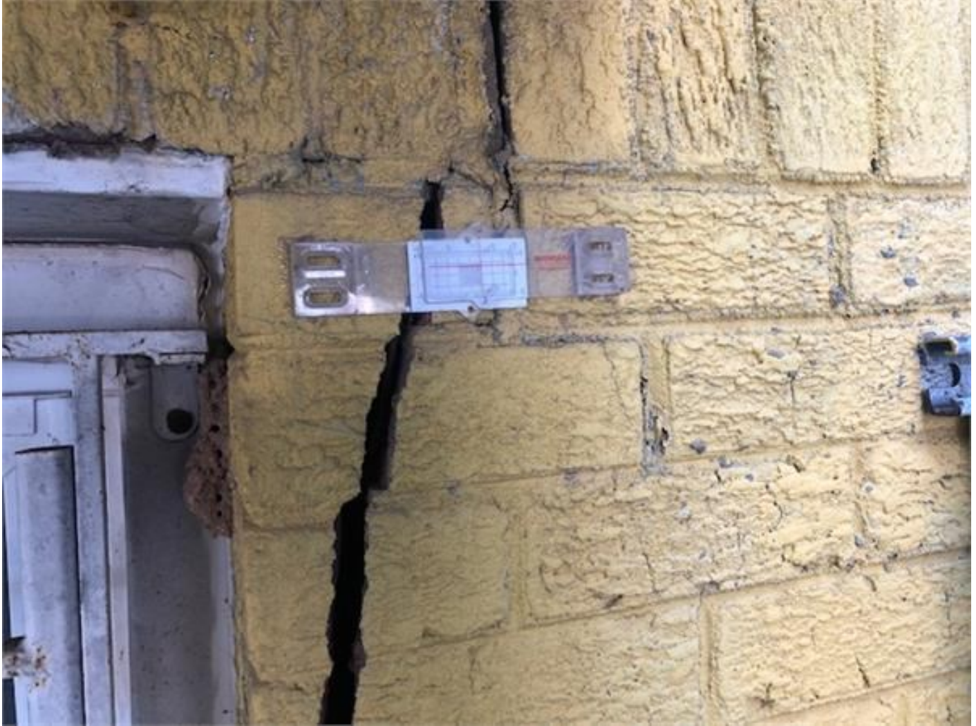
Fig 5. 770 Princeton Pl. NW@ Front underpinned wall.
