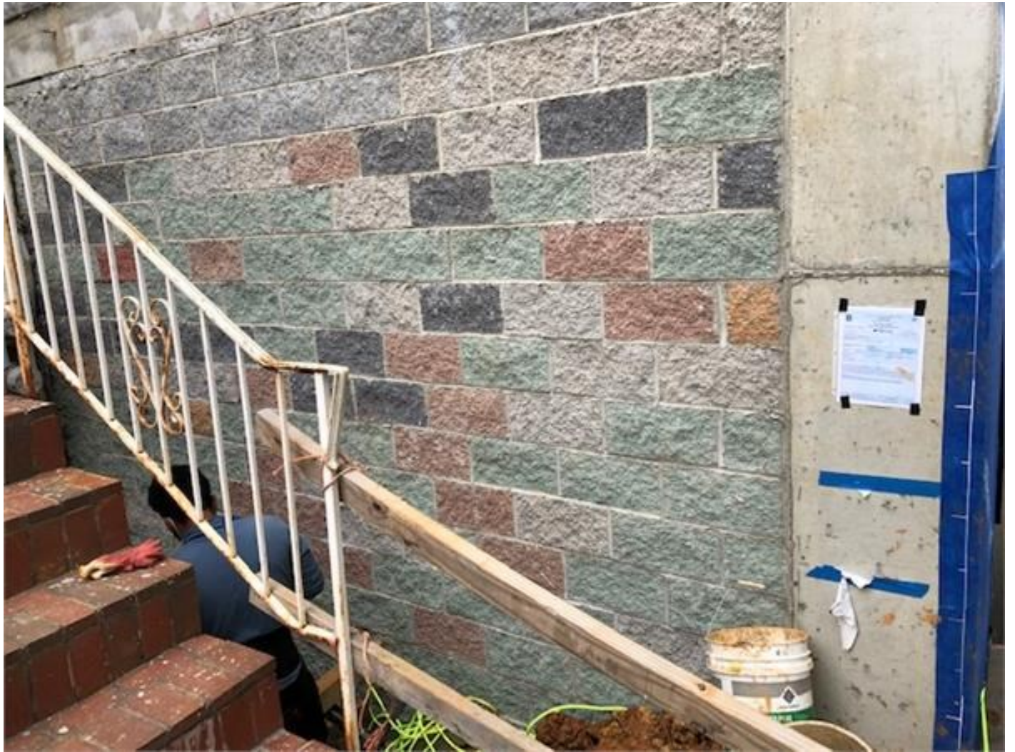
Fig 11. 770 Princeton Pl. NW@ detached adjacent wall on 3619 Georgia Ave NW.
