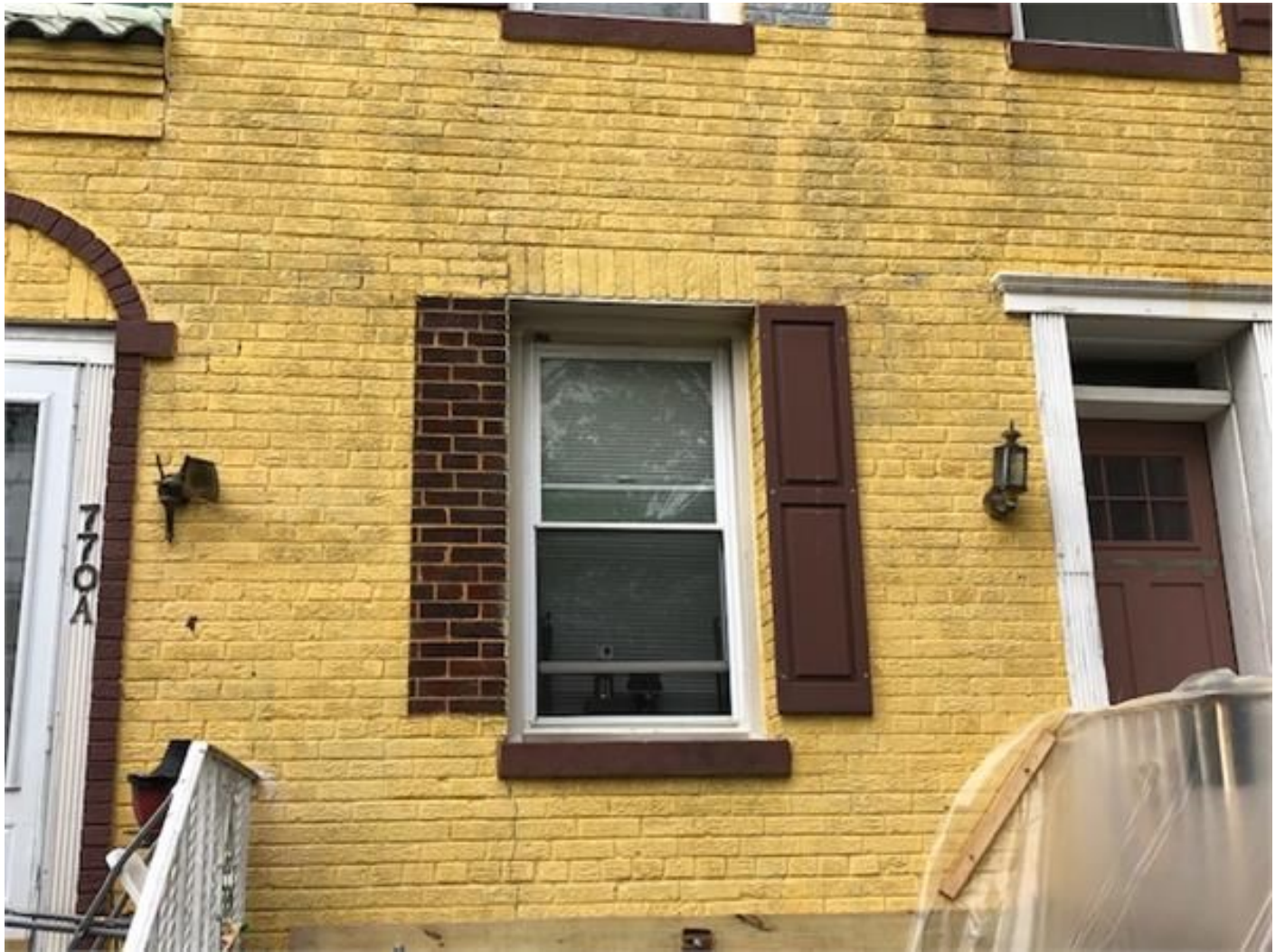
Fig 2. 770 Princeton Pl. NW@ Front underpinned wall.
