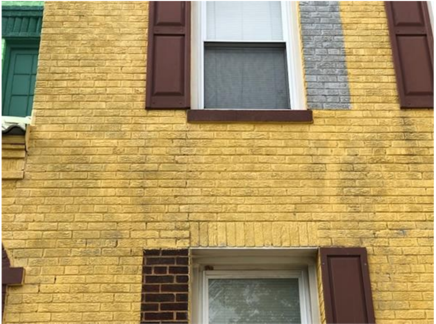
Fig 8. 770 Princeton Pl. NW@ Front underpinned wall.
