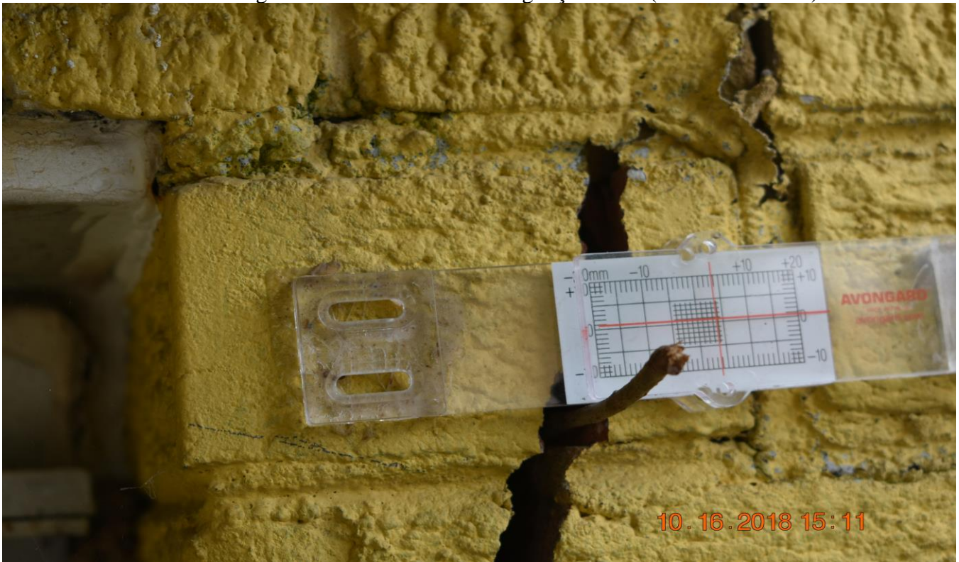
Monitor on right window corner of building façade wall (Taken 10/16/2018).
