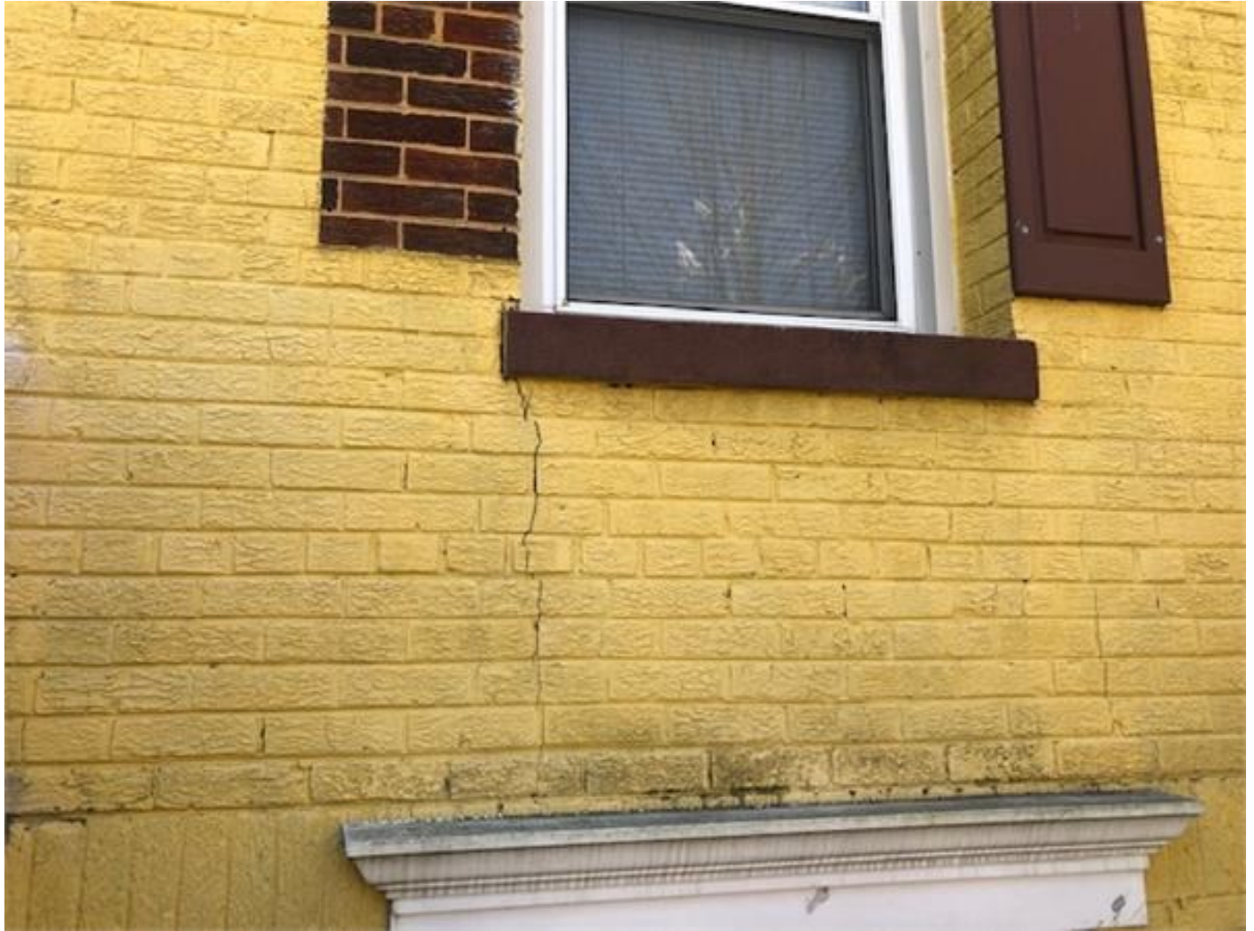
Fig 1. 770 Princeton Pl. NW@ Front underpinned wall.
