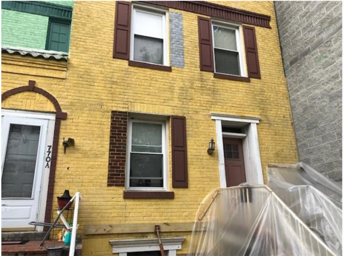
Fig 8. 770 Princeton Pl. NW@ Front underpinned wall.
