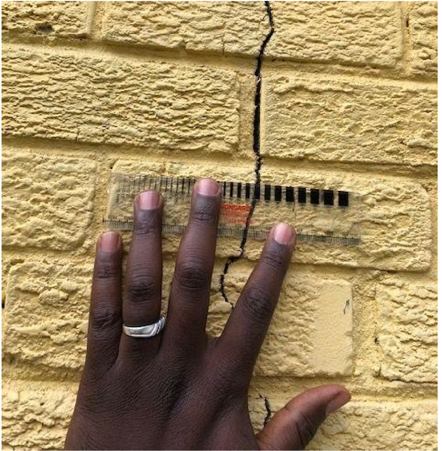
Fig 5. 770 Princeton Pl. NW@ Front underpinned wall.
