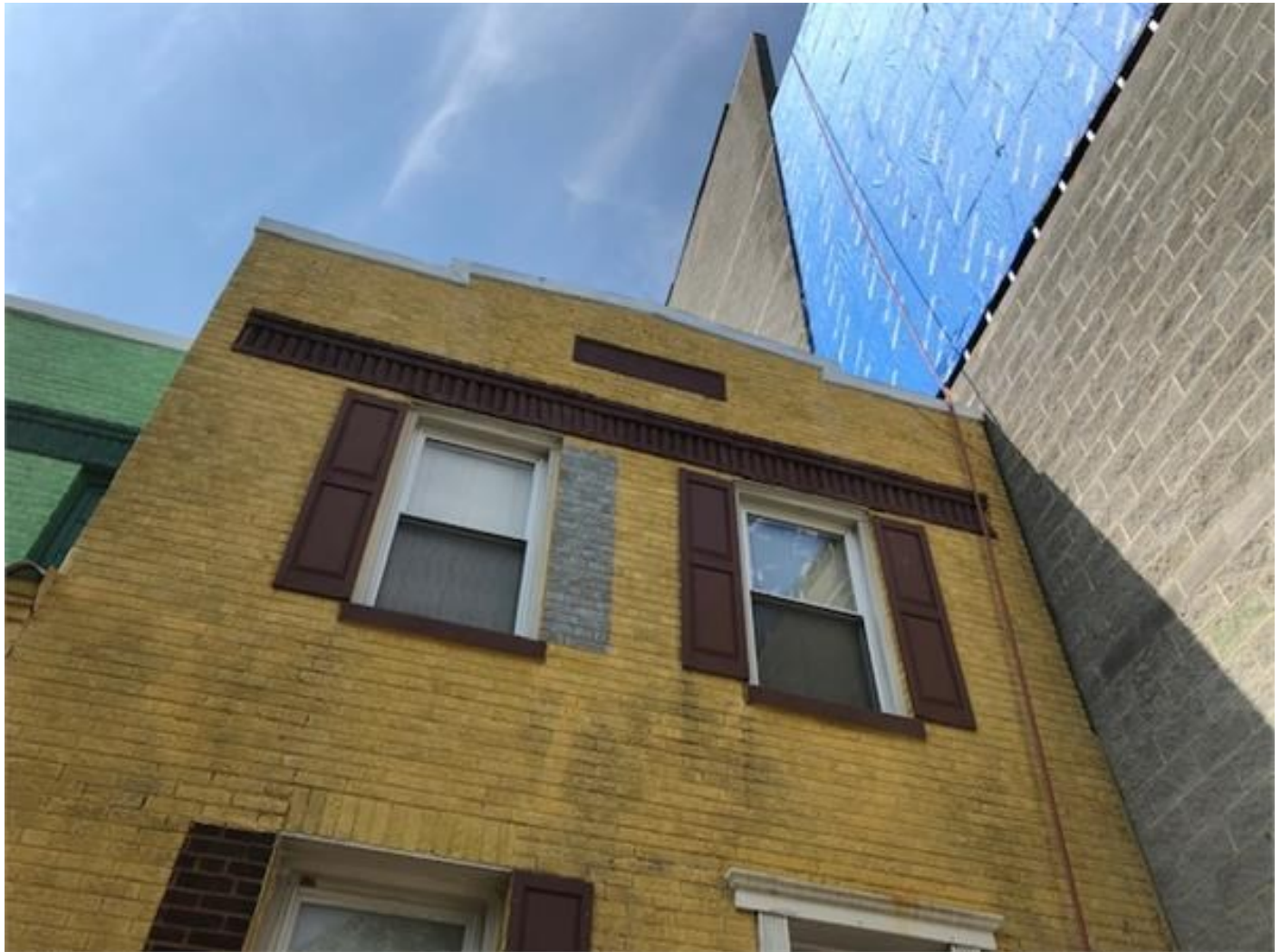
Fig 6. 770 Princeton Pl. NW@ Front underpinned wall.
