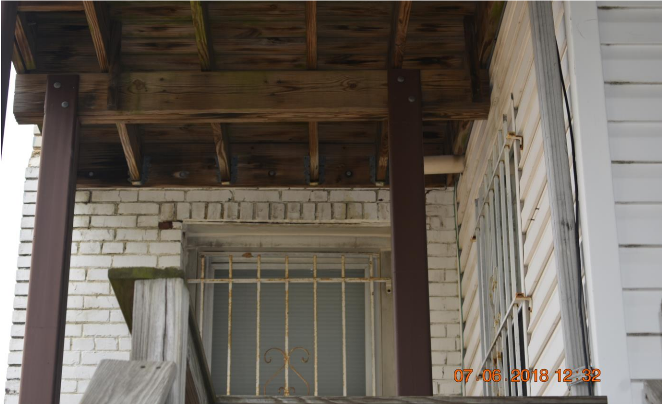
Rear deck post support on 7/6/2018
