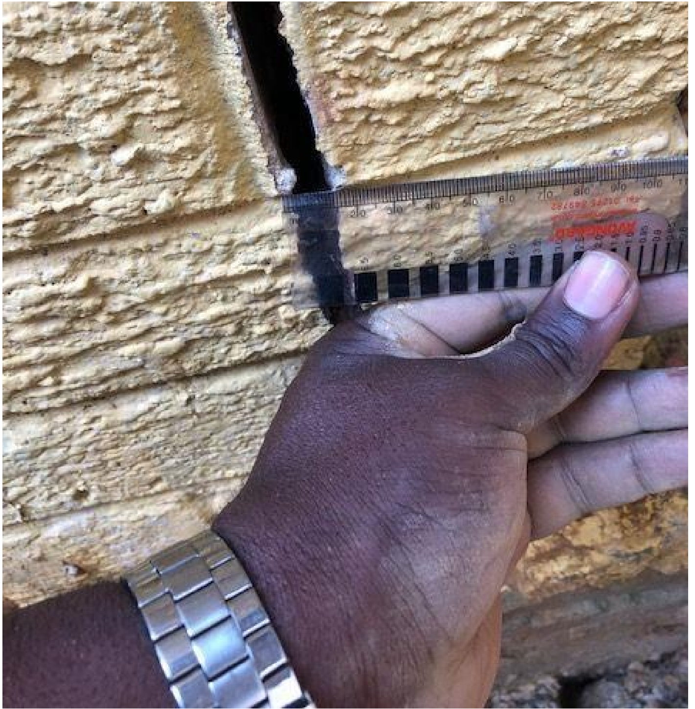
Fig 10. 770 Princeton Pl. NW@ Front underpinned wall.
