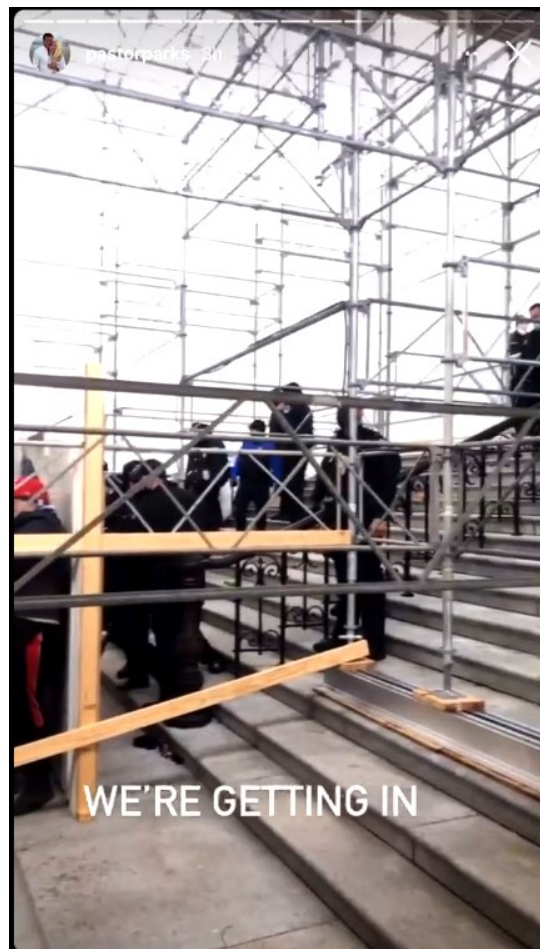
Image 4: Parks' Instagram Story on the Northwest Stairs underneath inauguration scaffolding.
