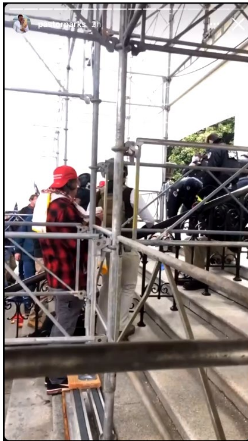
Image 5: Parks' Instagram Story on the Northwest Stairs underneath inauguration scaffolding.
