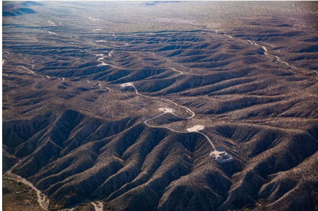
Figure 1: Aerial picture of new access roads and tower pad sites west of the San Pedro River, near Redrock Canyon. Photos taken by Archaeology Southwest with the support of a volunteer pilot and Lighthawk, a non-profit organization on November 13th, 2023, approximate coordinates: 32.17471, -110.34917.
